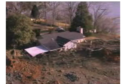
TVA Kingston Fossil Plant coal fly ash slurry spill Dec 22 2008 [http://www.tva.gov/emergency/ashslide_kingston.htm TVA
